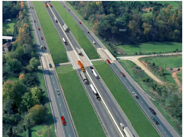
Figure 4: Ariel view of proposed I-81 Truck-Only Open Lanes in Virginia. Source: http://www.improve81.com/images/Interstate81_Final.jpg
